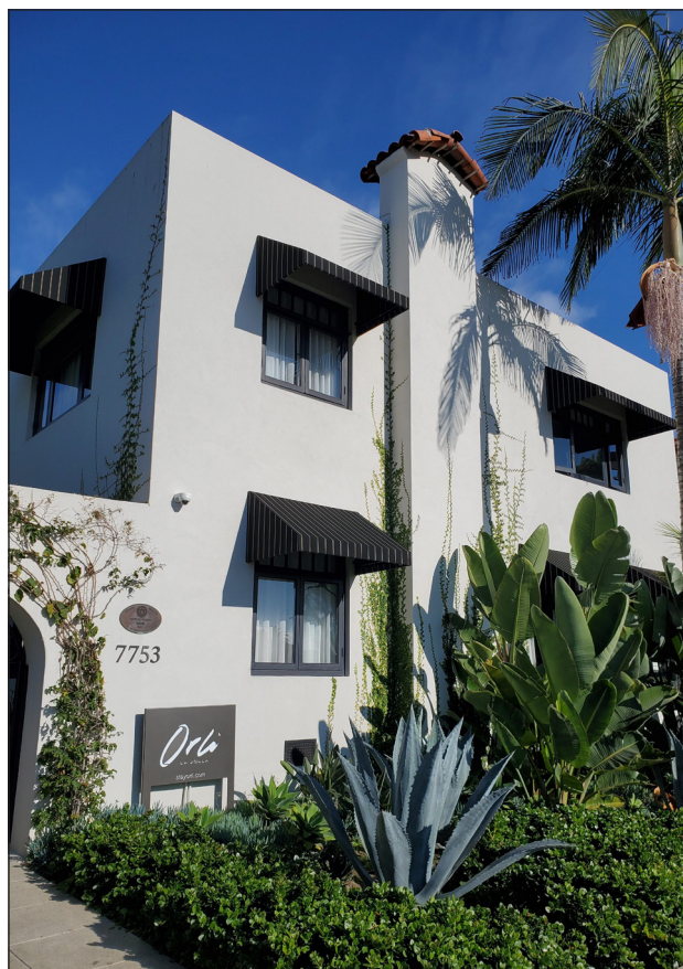
The Orli Hotel earned a Jewel Award for maintaining some of Irving Gill's signature architectural features.
